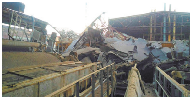
Approx. 3,500 thousand sq. m of the roofing structure collapsed in August 2017 at a workshop of the Crimean Titan (manufacturer of titanium dioxide)
