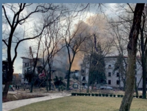
Drama Theater building after the air strike. According to various sources, in-between 500 and 1,200 people were hiding here. There may be 300 dead people under the rubble of the theater.
