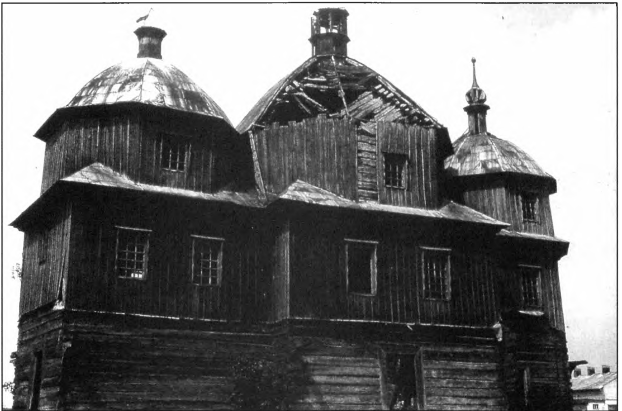
The Church of St. Michael the Archangel, built in the village of Verbytsia in 1886. Prior to Operation Wisla this Boiko-style wooden church featured three cupolas atop a three-tiered structure. After the local Ukrainian population was deported, the Poles closed the church and later converted it into a fertilizer warehouse. The floor and walls of the church are rotting from the chemicals, and the church is slowly falling into ruins.
