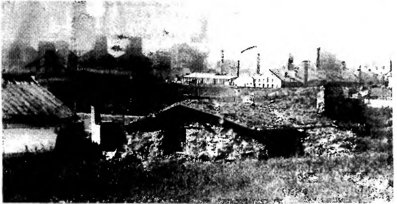
1.3 A zemlianka—a semidugout of earth and boards. Workers' housing up to the late 1890s.
