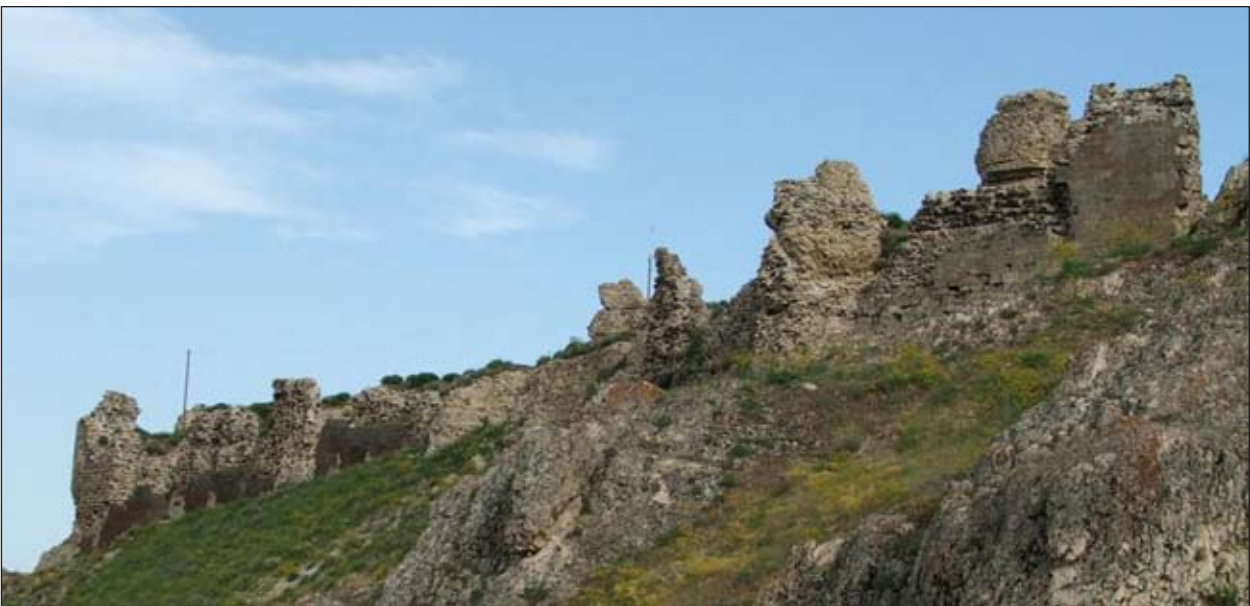
Fig. 8. The wall, adjacent to the north of the citadel (Phase II)
