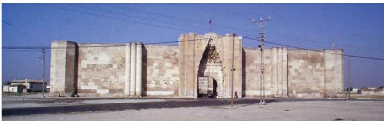
Fig. 2. Aksaray Sultan Hanı, Facade
