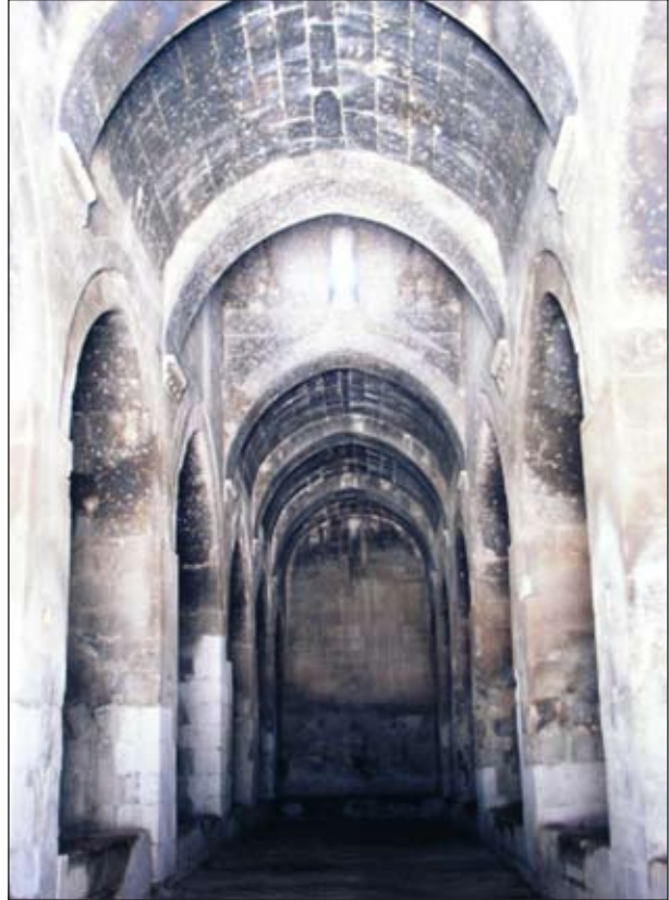
Fig. 6. Karatay Hanı, Interior of the Enclosed Section
