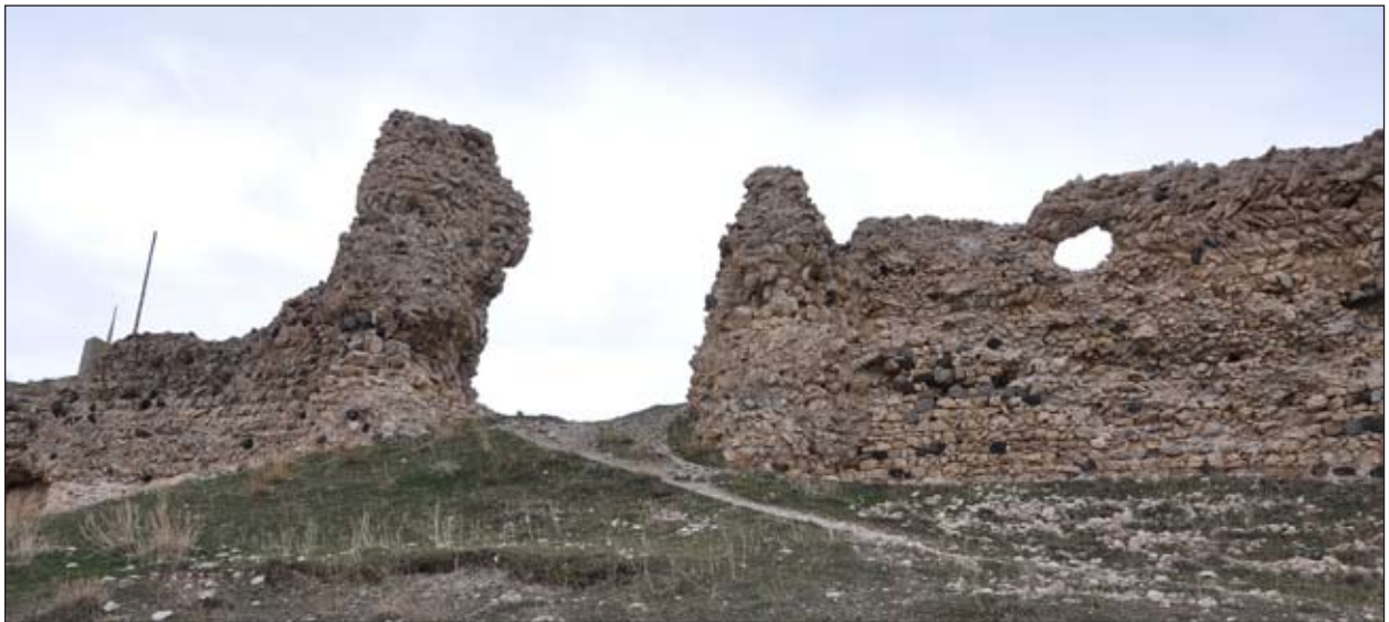
Fig. 6. The northern gate
